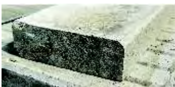
Beton vechi, beton
