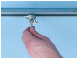
Systemfix is inserted into the C profile.
