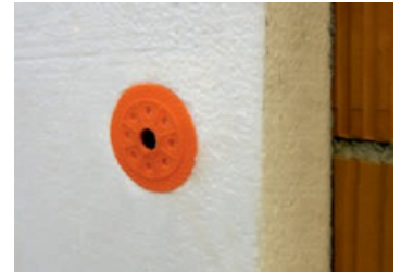
4 Diblu corect instalat
