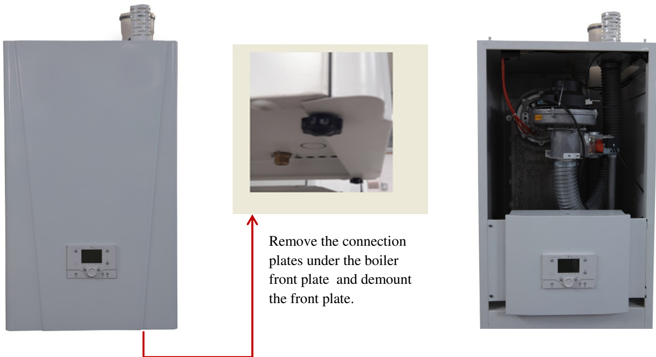
Visual-1: Demount of the Frount Plate
