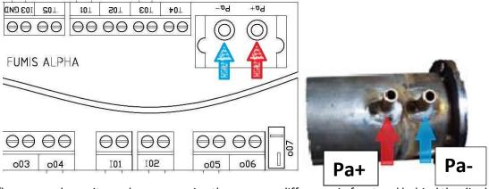
The air flow sensor bases its work on measuring the pressure difference in front and behind the diaphragm on the suction line of the boiler. The sensor itself is located directly on the control unit and is connected with the diaphragm using two silicone hoses for Pa + and Pa-. Based on the obtained measurement results, the control unit optimizes the combustion process in a way that controls the speed of the suction and exhaust fans.
