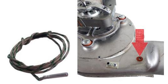
The sensor is intended for reading the temperature of the exhaust gases. The end of the sensor with the metal shield is placed in the required position on the exhaust fan housing as in the picture above. In the event that the fan is mounted on an adequate flange (in some versions of the boilers), the sensor is placed in the provided hole on the flange, it is necessary to ensure sealing between the sensor and the flange with a high temperature resistant silicone.
