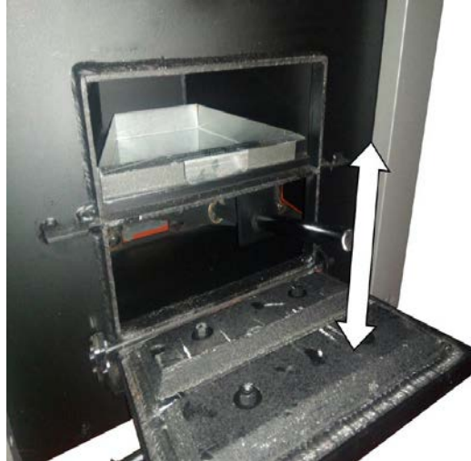
Figure 19. Cleaning the turbulators on boiler
