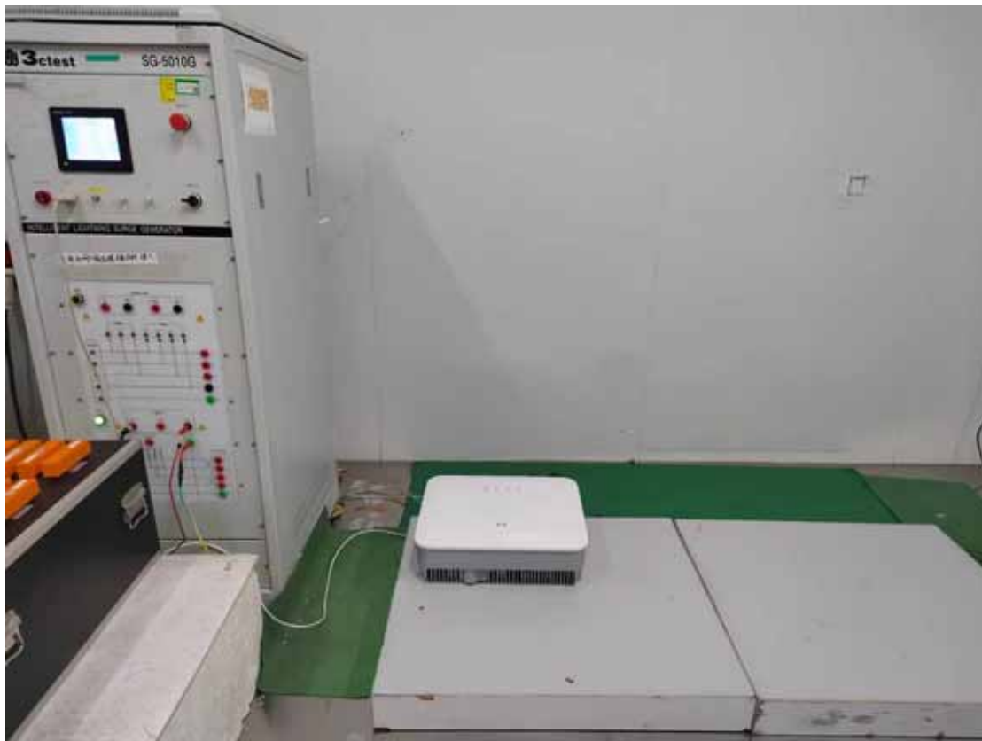
For Telecommunication port
