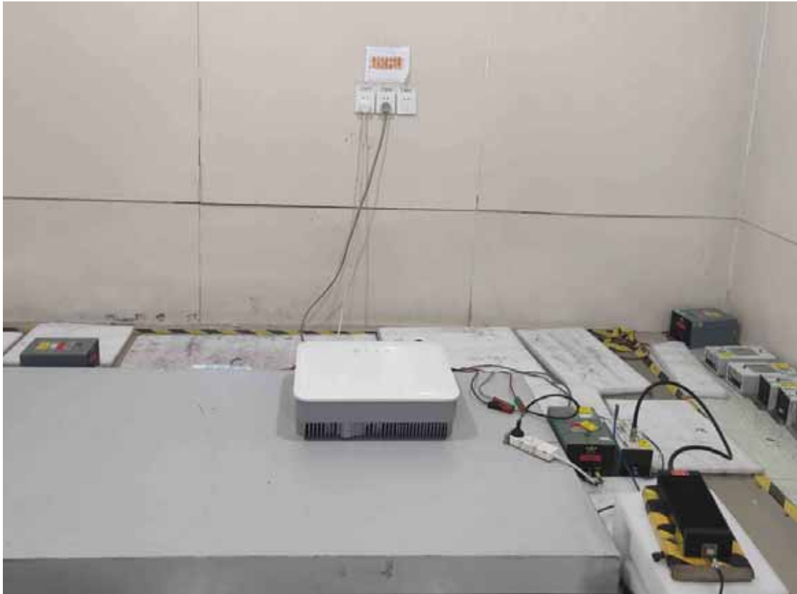
For Telecommunication port
