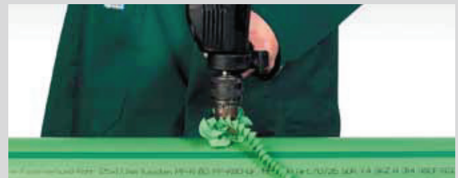
Drilling through the pipe wall
