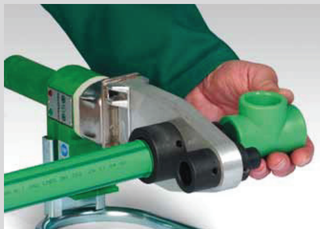
Heating-up of pipe and fitting
