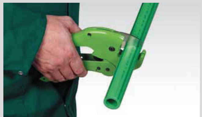
Cutting of the pipe
