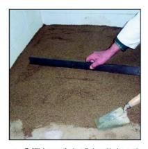
Pullfill the area for installation with dry sand and make it flat smoothly.
