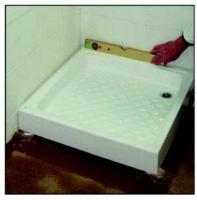
Do not give any additional slope since the shower trays have already a slope within. Protect the item until the end of construction work.
