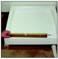
Place the shower in its location and fix the trap to waste water pipping. Always check the balance with the help of a water gauge.
