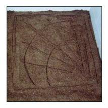
Place the shower tray temporarily to assembly position. The take it out, watch the traces on the sand. Add some sand if necessary for filling purposes.
