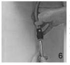
Connect the water supply hoses to the water supply stop handles on the wall using the crescent wrench. Do not turn the water supply handles on until the drain has been connected.
