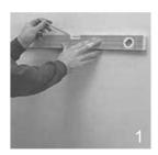
Use the torpedo level to get the most accurate positioning of the location and mark it with a pencil.
