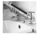
Once you have done all your tiling and flooring, you can seal where the basin is in contact with the wall Check all of the parts correctly and finish the installation
