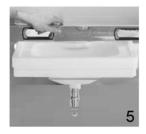
Hang the sink on the bracket to mount it onto the wall. Place the torpedo level on the front lip of the sink to make sure that the sink is level.
