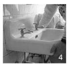
Hang the sink on the bracket to mount it onto the wall. Place the torpedo level on the front lip of the sink to make sure that the sink is level.
