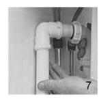
Make the Pop-Up waste connect the P-Trap by all of the plastic and rubber washers. Fit the trap to the basin waste.
