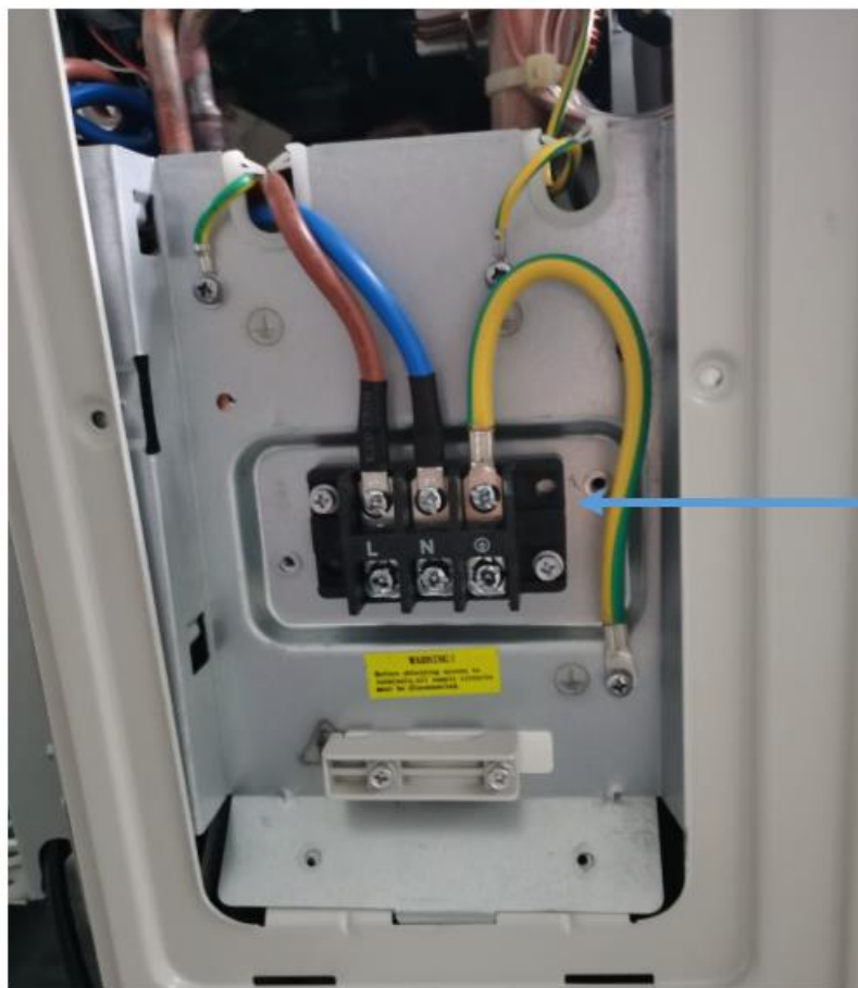
Figure 5-1.4: Power Supply Terminals
