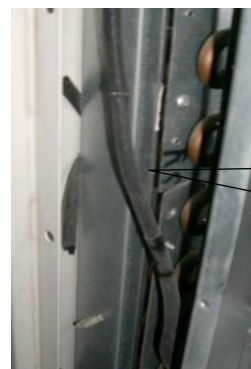
T4 sensor is worn out and connected with sheet metal
