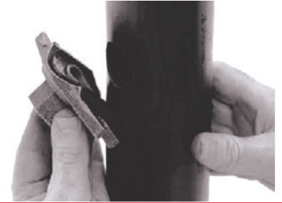
3. Gasket Installation
