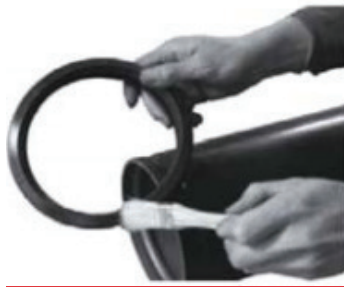
2. Lubricate Gasket
