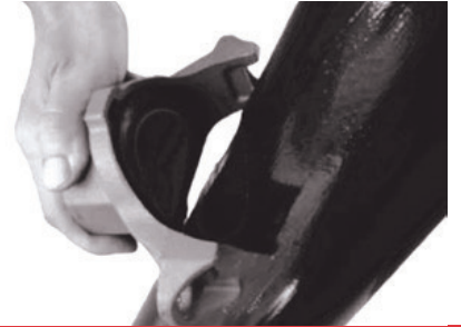
3. Gasket installation
