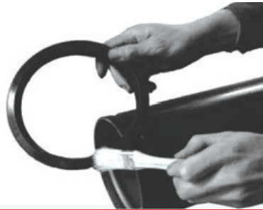
2. Lubricate Gasket
