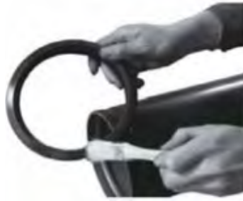
2. Lubricate Gasket
