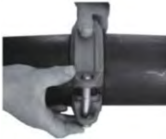
5. Housing Installation
