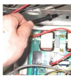
Figure 4-4.5: Measuring resistances between compressor terminals and ground
