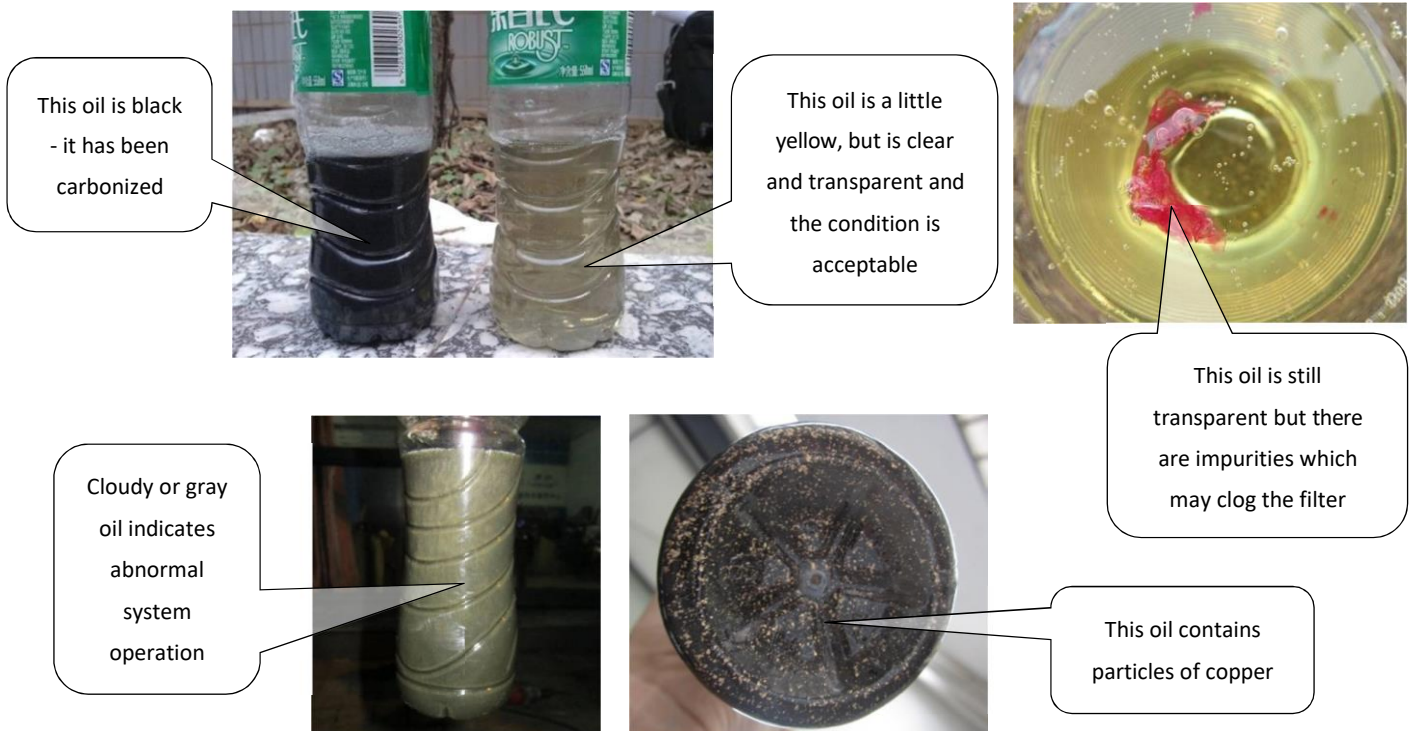
Figure 4-4.11: Inspecting compressor oil
