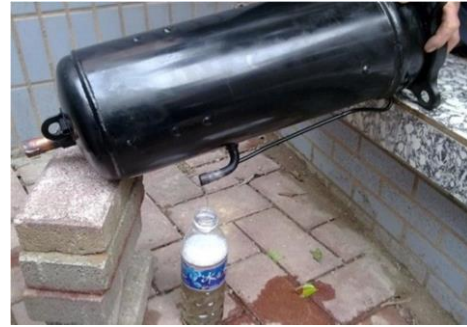
Figure 4-4.10: Draining oil from a compressor
