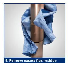
• Flux residue **must** be removed so the joint can be properly inspected, and tested.
