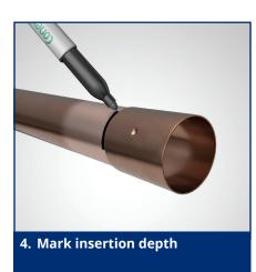
• Mark the correct insertion depth on the tube.
