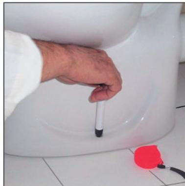
**5** Bring the wc pan temporarily to assembly position. Mark the holes on both sides on to the finished floor.
