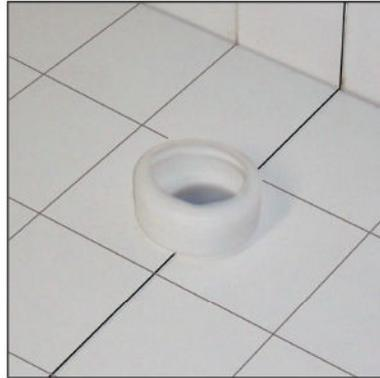
**2** Place the eccentric trap adapter to its location inside the waste water outlet.
