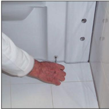
**13** Place the wc pan to final assembly position. Slide assembly screws through plastic bushes and screw to main mounts at both sides of the WC pan.
