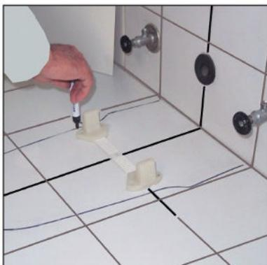
**7** Join the markings at the 4th figure horizontally. Intersect it also with the vertical axis drawn before. Overlap the strip's "+" sign with the intersection of axis on the floor. Now, mark the holes of the main mounts on the strip.
