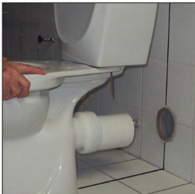
**4** Slide the eccentric trap adapter to the outlet of the wc pan. Calculate the gap, which is needed for extension for the waste piping.
