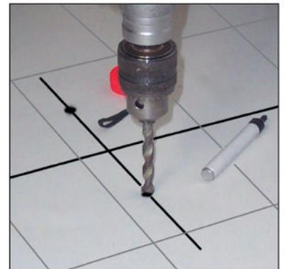
**6** Drill the marked points with suitable drill bits and insert the raw plugs.
