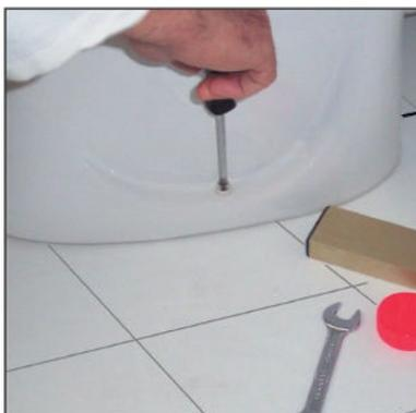
**7** Place the wc pan to its final position and fix it by using its original assembly kit.
