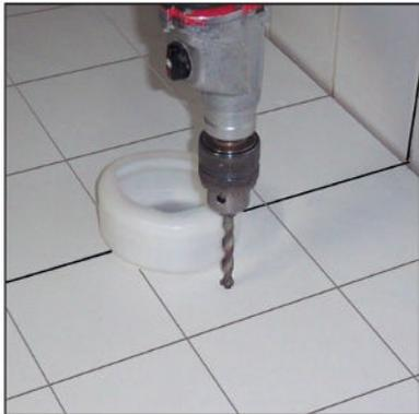
**4** Drill the marked points with suitable drill bits and insert the raw plugs.
