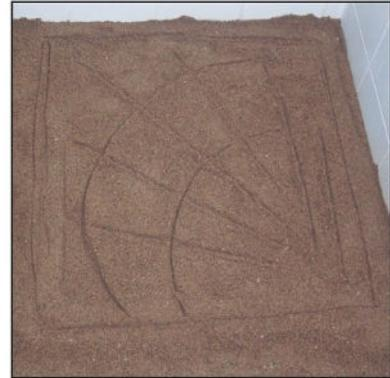
**3** Place the shower tray temporarily to assembly position. The take it out, watch the traces on the sand. Add some sand if necessary for filling purposes.
