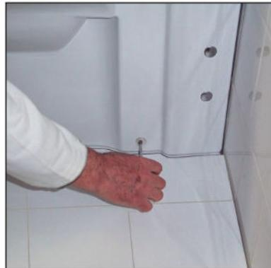
**14** Place the wc pan to final assembly position. Slide assembly screws through plastic bushes and screw to main mounts at both sides of the WC pan.
