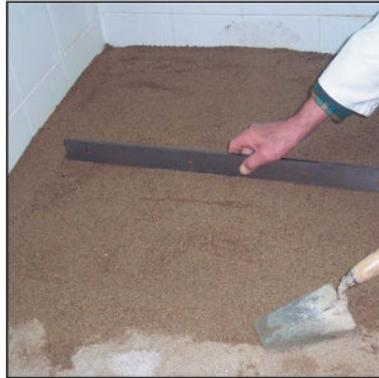
**2** Fullfill the area for installation with dry sand and make it flat smoothly.
