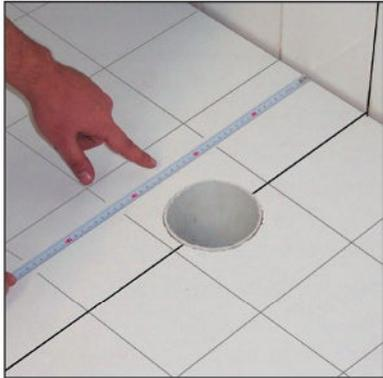
**1** Set the distance between the outlet of the wc pan and the finished wall. Prepare the waste water outlet on the floor.
