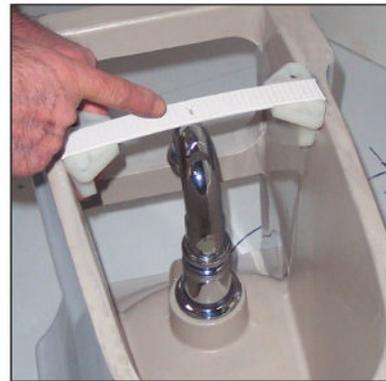
**6** Place the main mounts on the strip. Check the gap now with strip; mounts on it. The length of the strip may neither long nor short.
