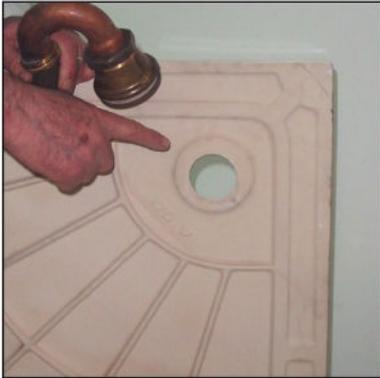
**1** Install the trap on to the waste hole of shower tray.
