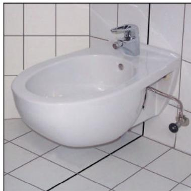
**5** Test the wc pan for a possible leakage. Silicone based pastes may be applied on the joining edges of the ceramic and finished wall for a better tightness and aesthetic view.
