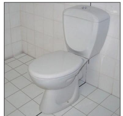
**9** Test the wc pan for a possible leakage. Silicone based pastes may be applied on the joining edges of the ceramic and finished wall for a better tightness and aesthetic view.
