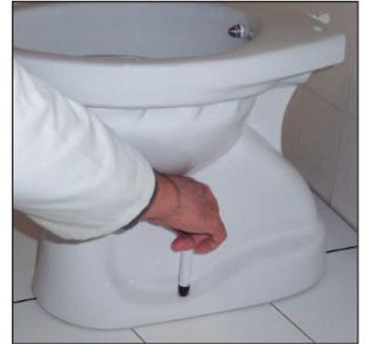
**3** Bring the wc pan temporarily to assembly position. Mark the holes on both sides on to the finished floor.
