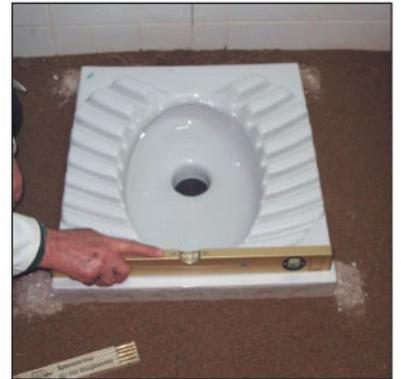
**3** Fix the squatting pan at four corners with a rich mixture of cement. The joint filling material for ceramic tiles will be quite enough for final fixing of the squatting pan.
