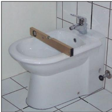
**4** Place the bidet temporarily to assembly position. Use the assembly holes as reference points and mark the projections on the finished floor.
