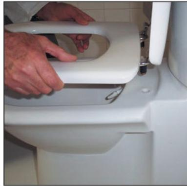
**14** Each WC pan has its own seat cover. Thus, place the seat cover with its hinges on it, by sliding the screws through installation holes on the pan.
