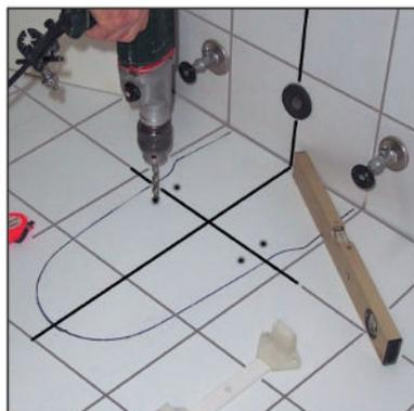
**8** Drill the marked points and insert the plugs.
