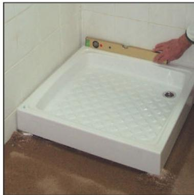
**5** Do not give any additional slope since the shower trays have already a slope within. Protect the item until the end of construction work.
