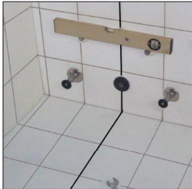
**1** After installation of the carriage bracket; the waste water outlet and interval tap inlets are prepared and proceed on tile works.
