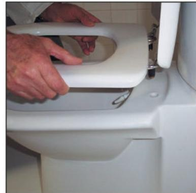
**15** Each WC pan has its own seat cover. Thus, place the seat cover with its hinges on it, by sliding the screws through installation holes on the pan.
