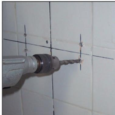
**5** Place the (+) sign on the adjustment with the intersection point, mark the holes of the mounts on both sides. Drill the marked points with suitable bits and insert raw plugs.
