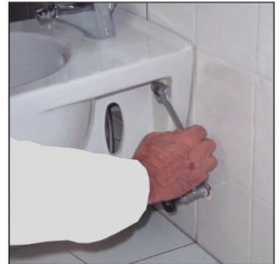
**3** Push the bidet forward to assembly position. Slide the syphon through the waste water outlet. Fix the assembly nuts of the bidet.
