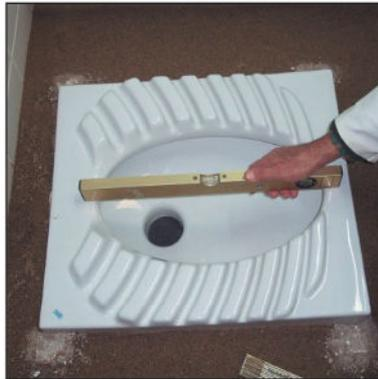
**2** The squatting pan must be installed on dry sand like shower trays. Check out that there will be no void under the pan, thus add enough sand to keep the tightness.
