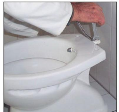
**6** Connect hidden lustration pipe and connection adapter with 3/8" flexible pipe on WC Pan.
