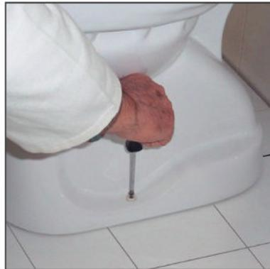
**5** Place the wc pan to its final position and fix it by using its original assembly kit.
