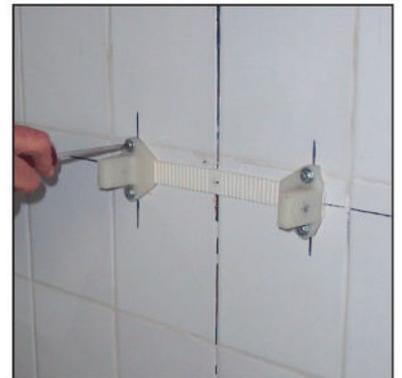
**6** Fix the stick with assembly mounts on it.
