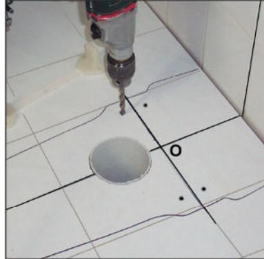
**11** Overlap the strip's "+" sign with the intersection of axis on the floor. Now, mark the holes of the main mounts on the strip. Drill them.
