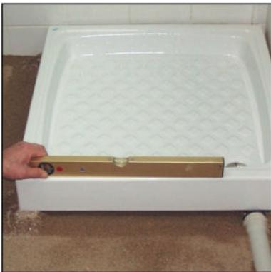
**4** Place the shower in its location and fix the trap to waste water piping. Always check the balance with the help of a water gauge.
