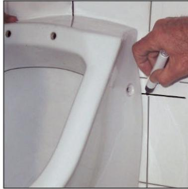
**2** Place the urinal temporarily to assembly position, mark the projection of the product and assembly holes intersect vertical and horizontal axis.
