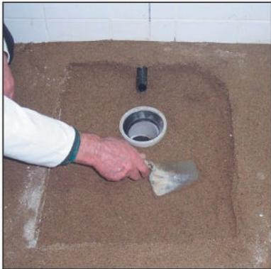
**1** First, prepare the infrastructure, trap, flashing piping, etc.
