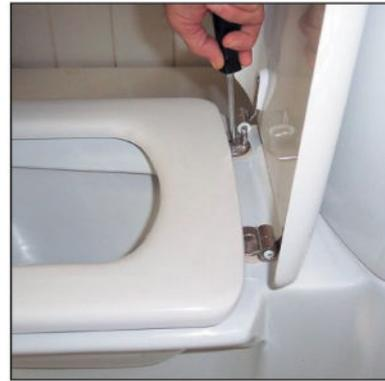
**15** Use a simple cross-head screwdriver to tighten the seat cover.
