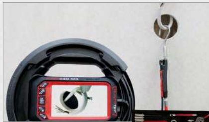
Cavity wall inspection
