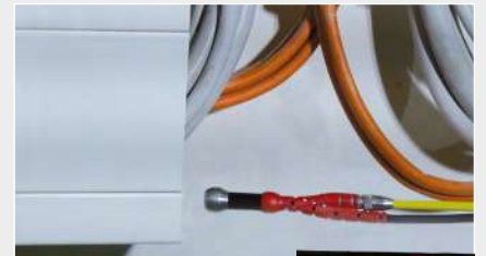
Shafts and underfloor ducting
