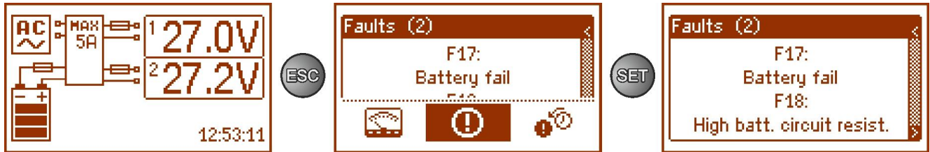
Fig. 19. LCD screen – current failures of PSU.
